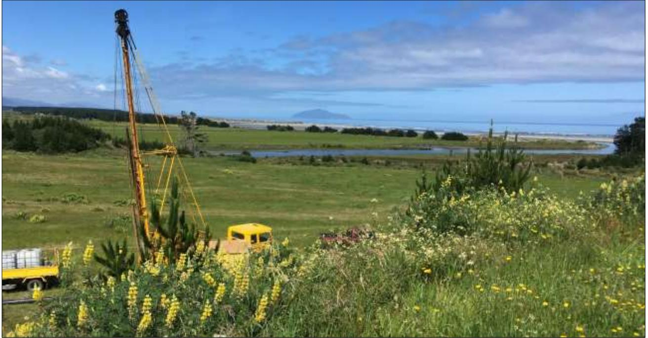
**Figure 6. The Neville Webb Welldrilling cable-tool rig drilling the new Well. View southwest toward the Ohau River, and coastline to the west.**
